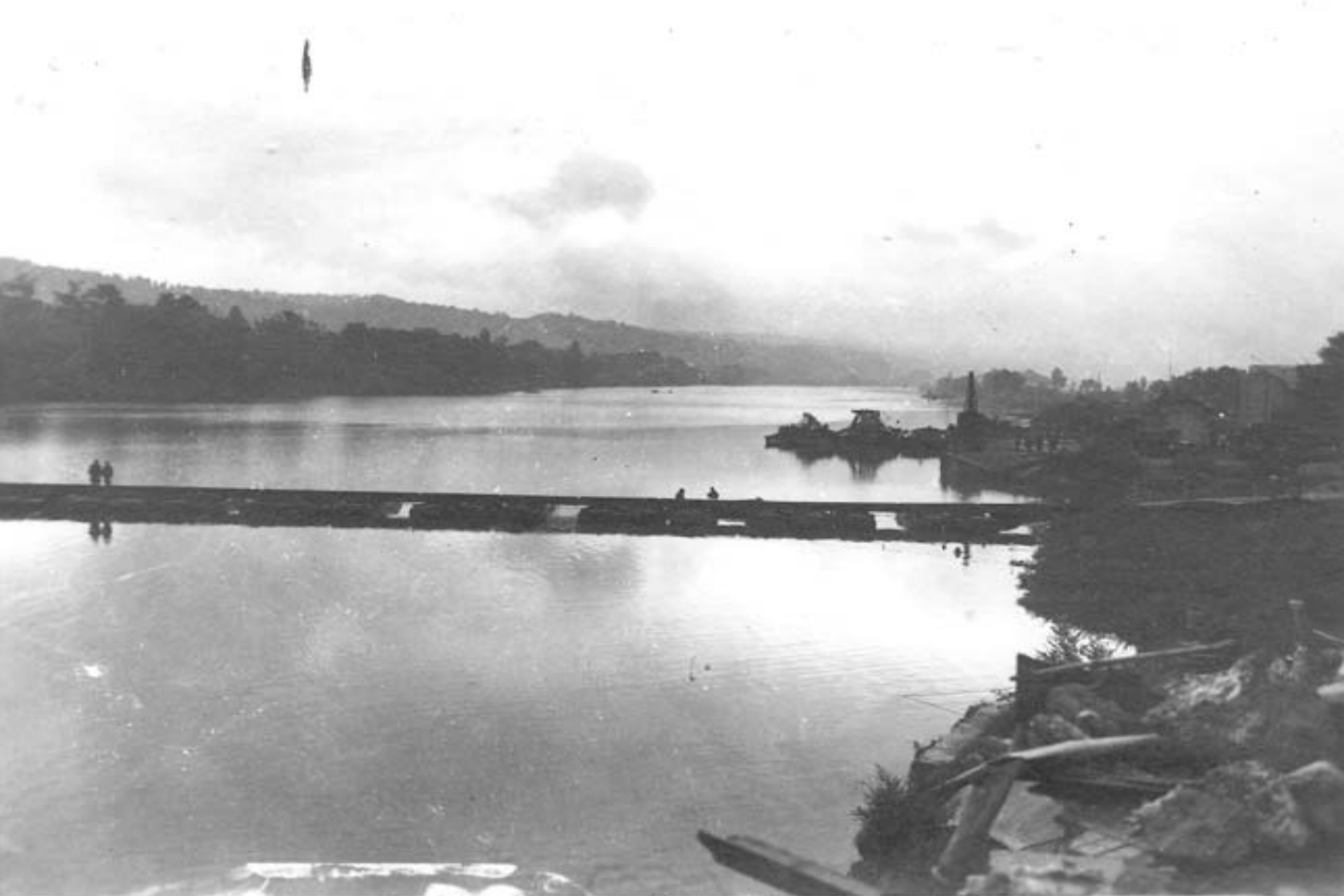
Views of 720' Treadway Bridge, Seine Riv., Meulan, France; constr. by 82 Engr. C Btn. 29 Aug '44
