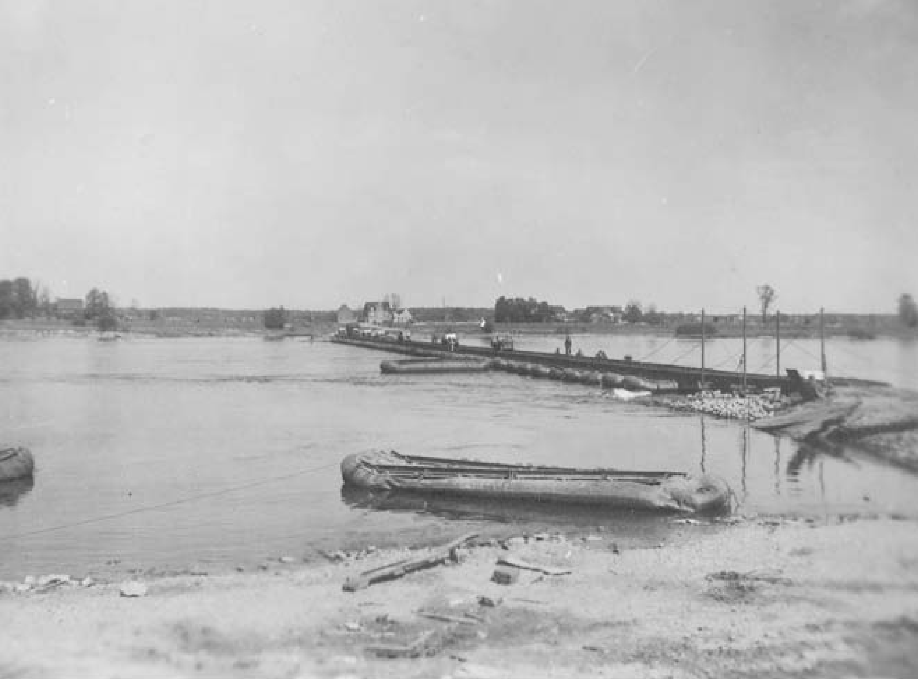
Treadway Bridge Elbe River Vicinity Barby, Germany - 20 April '45
