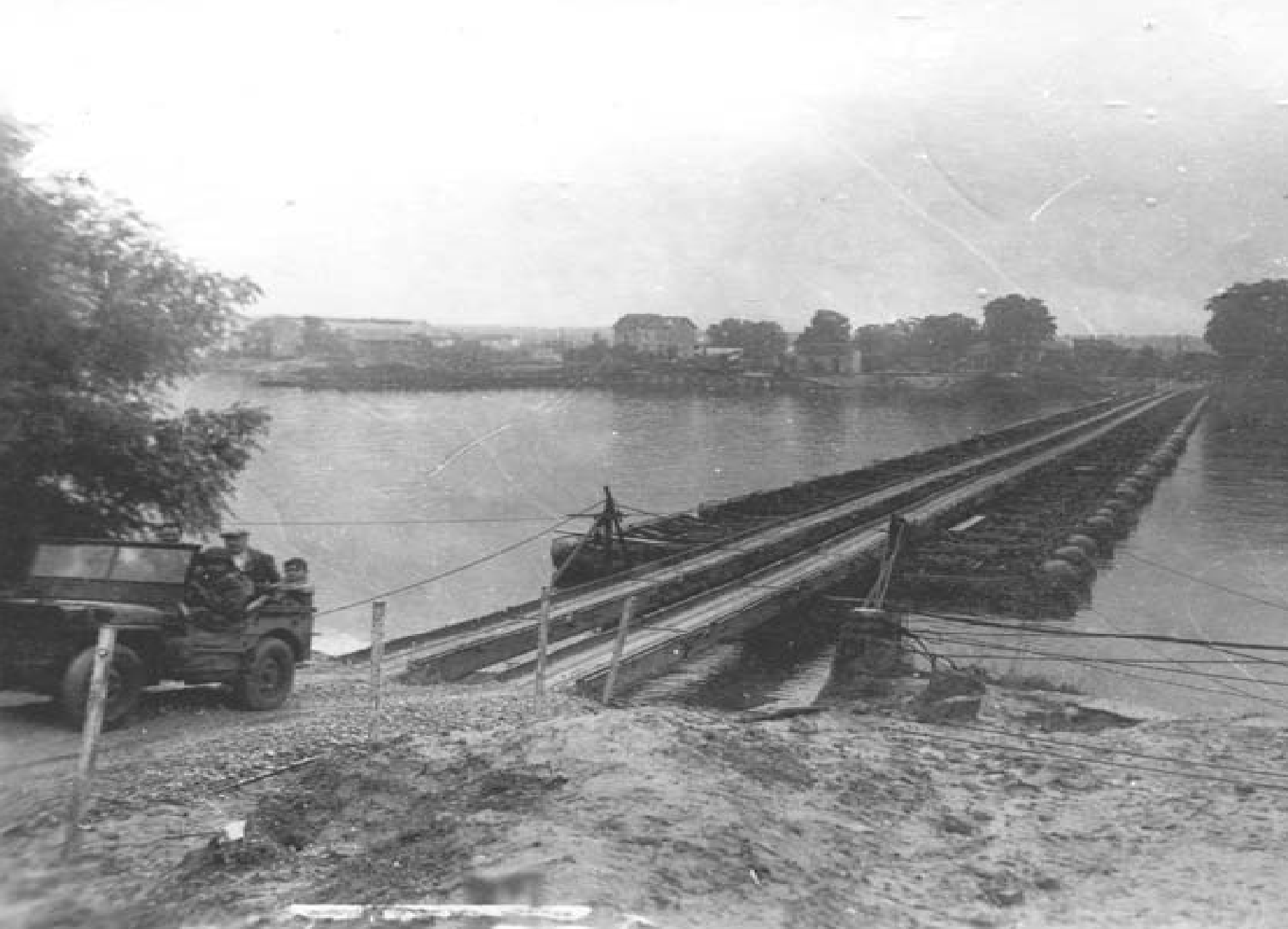
Views of 720' Treadway Bridge, Seine Riv., Meulan, France;
