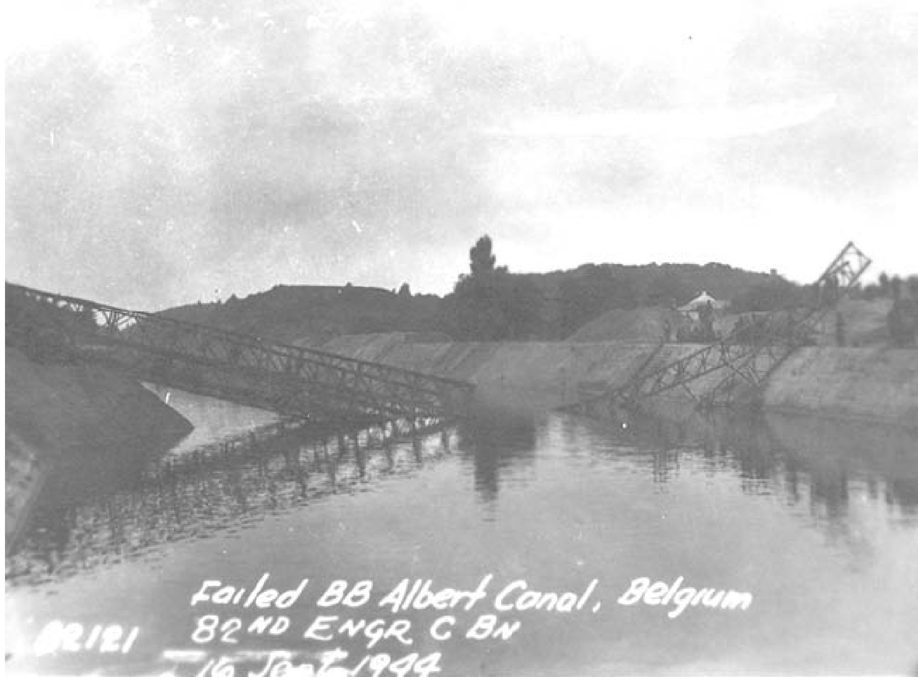
Failed panel, BB Albert Canal, Belgium 82nd Engrs. C BN 16 Sept. '44
